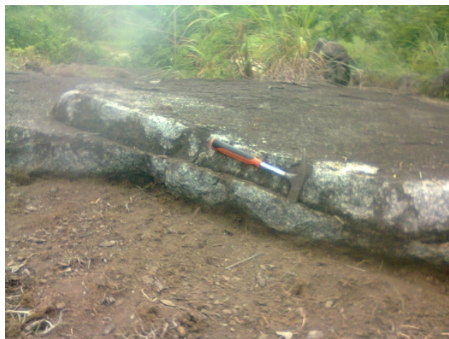
Fig. 4. Sheet/Exfoliation joints in granites around Igarra/Somorika
